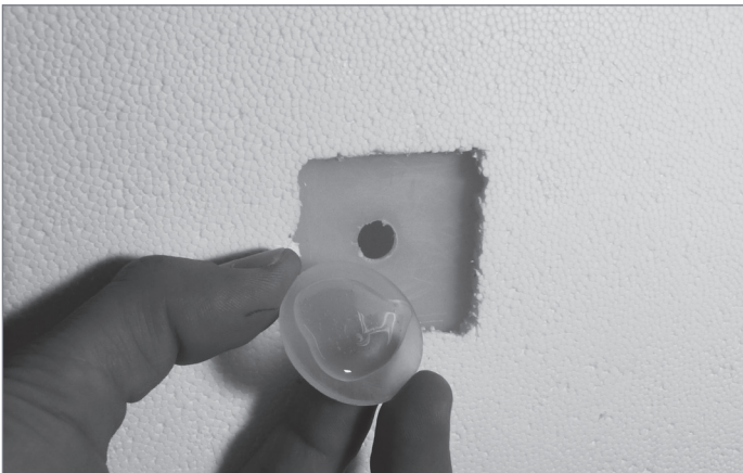
5. Coat the plastic discs with PP-glue with help of hot-melt gun (double hole size). Use only original PP glue and don't mix it with other glues!
