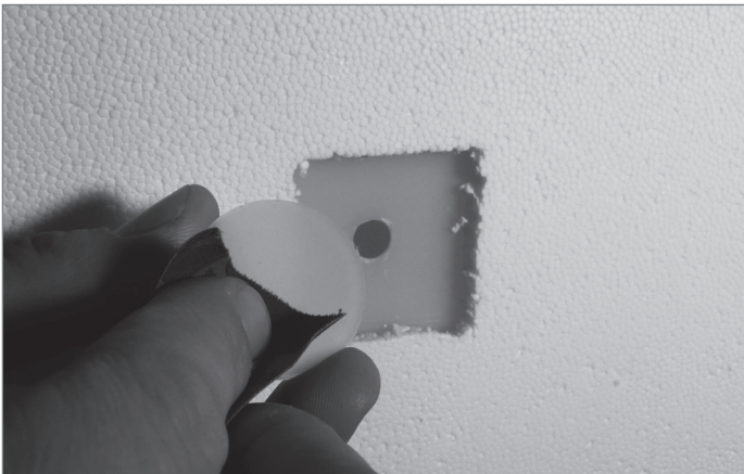
3. Roughen both glue areas with abrasive paper
