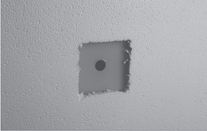
1. Clean the damaged areas
