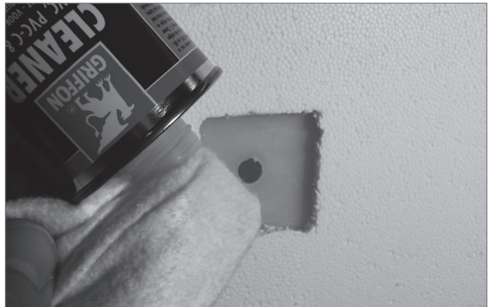
4. Clean both glue areas with acetone or provided cleaner
